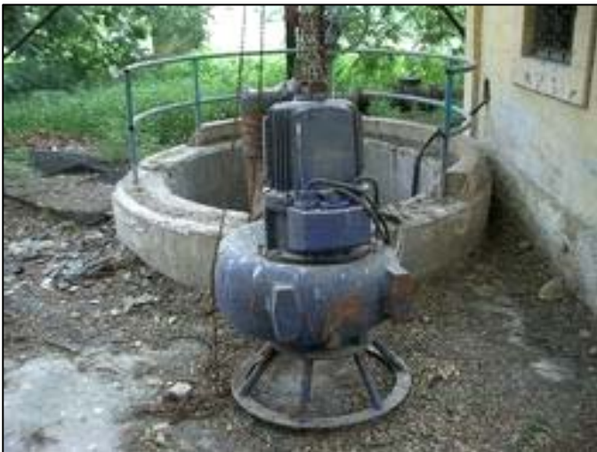
Photo 33.2.11 Submersible Pump of Jamila Pumping Station
