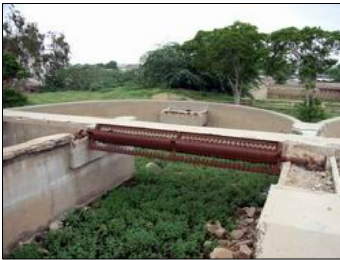
Photo 33.2.26 Oxidation Ditch (North Karachi TP, abandoned)
