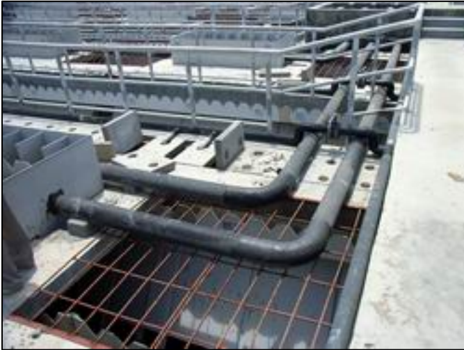
Photo 33.2.28 Inlet Pipes and Distribution Box of UASB (TP of PTA)
