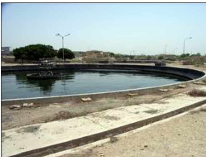
Photo 33.2.20 Final Settling Tank (TP-1, in May 2006)
