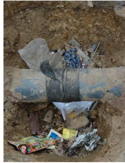
Photo 33.1.4 4" PVC Plugging by Rubber Tube
