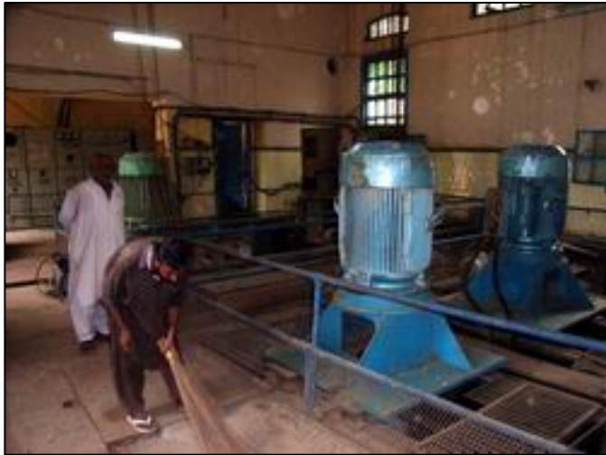
Photo 33.2.10 Vertical Pumps of Jamila Pumping Station
