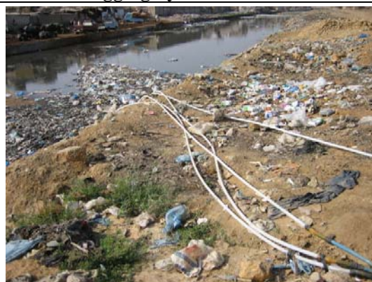
Photo S32.1.4 Piping for Illegal Connections across the Canal
