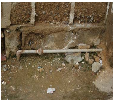
Photo S32.1.1 3/4" GIP Service Connection
