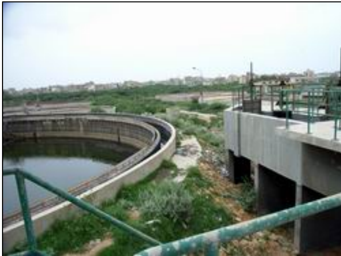
Photo 33.2.18 Primary Settling Tank (TP-2, in August 2006)
