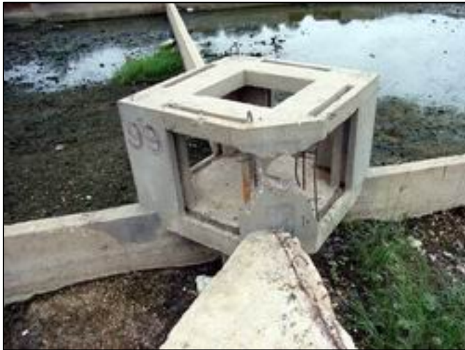
Photo 33.2.21 Sludge Distribution Box (TP-2, August 2006)
