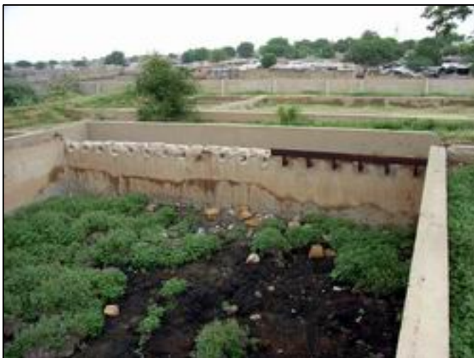
Photo 33.2.27 Final Settling Tank (North Karachi TP, abandoned)
