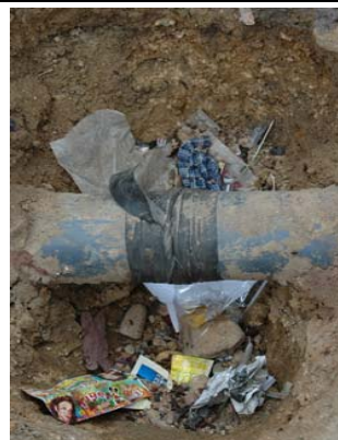
Photo S32.1.2 4" PVC Plugging by Rubber Tube
