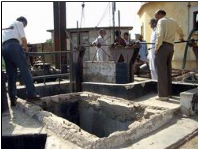
Photo 33.2.5 Screen Facility of Pumping Station PS-2 in Korangi
