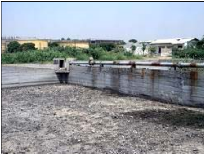
Photo 33.2.22 Sludge Distribution Pipe and Box (TP-1, September 2006)
