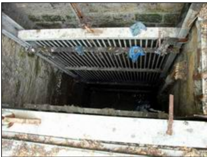
Photo 33.2.9 Screen Facility of Jamila Pumping Station
