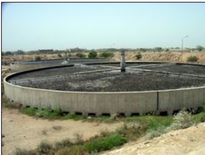
Photo 33.2.19 Trickling Filter (TP-1, in May 2006)
