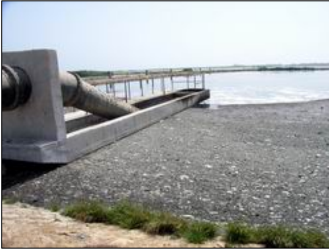
Photo 33.2.24 Inlet to Anaerobic Pond (TP-3, in September 2006)
