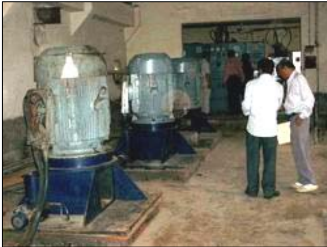
Photo 33.2.14 Vertical Type Pumps of Chakiwara Pumping Station
