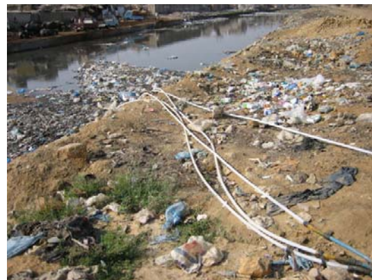
Photo 33.1.6 Piping for Illegal Connections across the Canal
