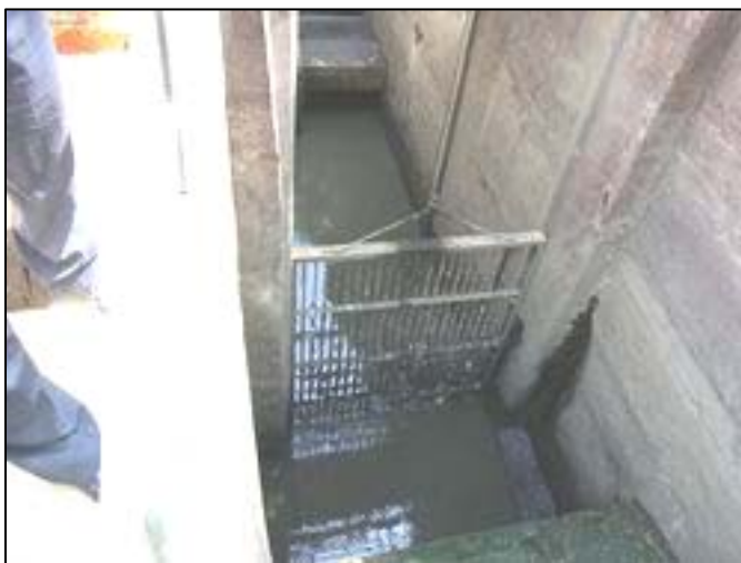
Photo 33.2.1 Screen Facility of Clifton Pumping Station
