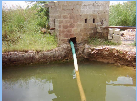
At the bulk pumping station of Hub, water constantly overflows forming a pool, siphoning pipe is in place, a hydrant is in operation since more than 15 years.
