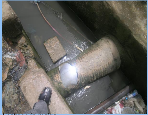
Leakage in mains
