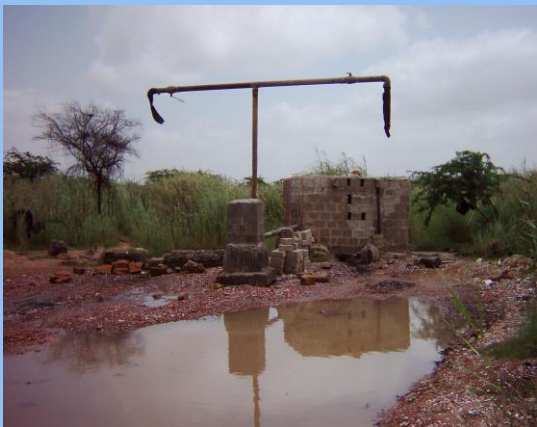
At the bulk pumping station of Hub, water constantly overflows forming a pool, siphoning pipe is in place, a hydrant is in operation since more than 15 years.
